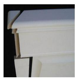
You will require a table saw to cut the stile down straight on one side. The stile should sit about a quarter inch in from the bottom of the Upper Rail; this will give it a more finished look.
