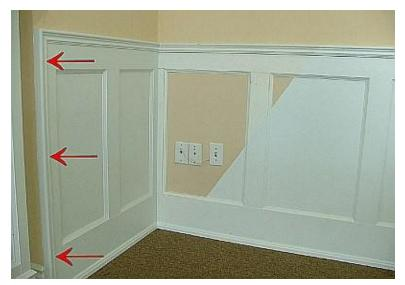
Making a Return using the Top Rail is the best method of finishing wainscoting mid-way on a wall. When you get to where you want to end the Wainscoting, you simply miter the various pieces of the kit so that they create a 90 degree angle facing towards the wall as shown in the image.
