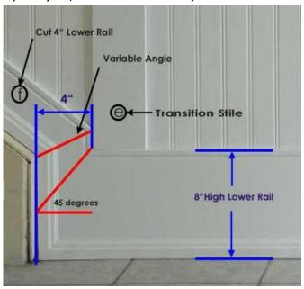
3) Note the position of the Transition Stile (e) and both the top and bottom transitions in the different pictures included in this instructional. The Bottom Transition is placed next to the stile (e) whereas the Top Transition is placed above the stile (e). This is done in order to accommodate the stringer without interfering with; or protruding into the panel. Using this technique also prevents odd "L" shaped panels which are difficult to cut and especially difficult to shape using a router.
