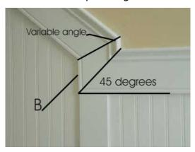
4)The next part to consider is the small transition (b) on the Top Rail between the horizontal installation and the diagonal stair Installation. Follow the same guidelines set for the Lower Transition described in Step 2. The difference here is that the Top Rail is installed at full height and should not be cut down in height. Remember that the variable angle will remain the same for both the top and the bottom of the installation.
